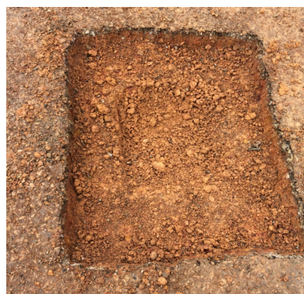
Figure 2. Open trench for sample removal
